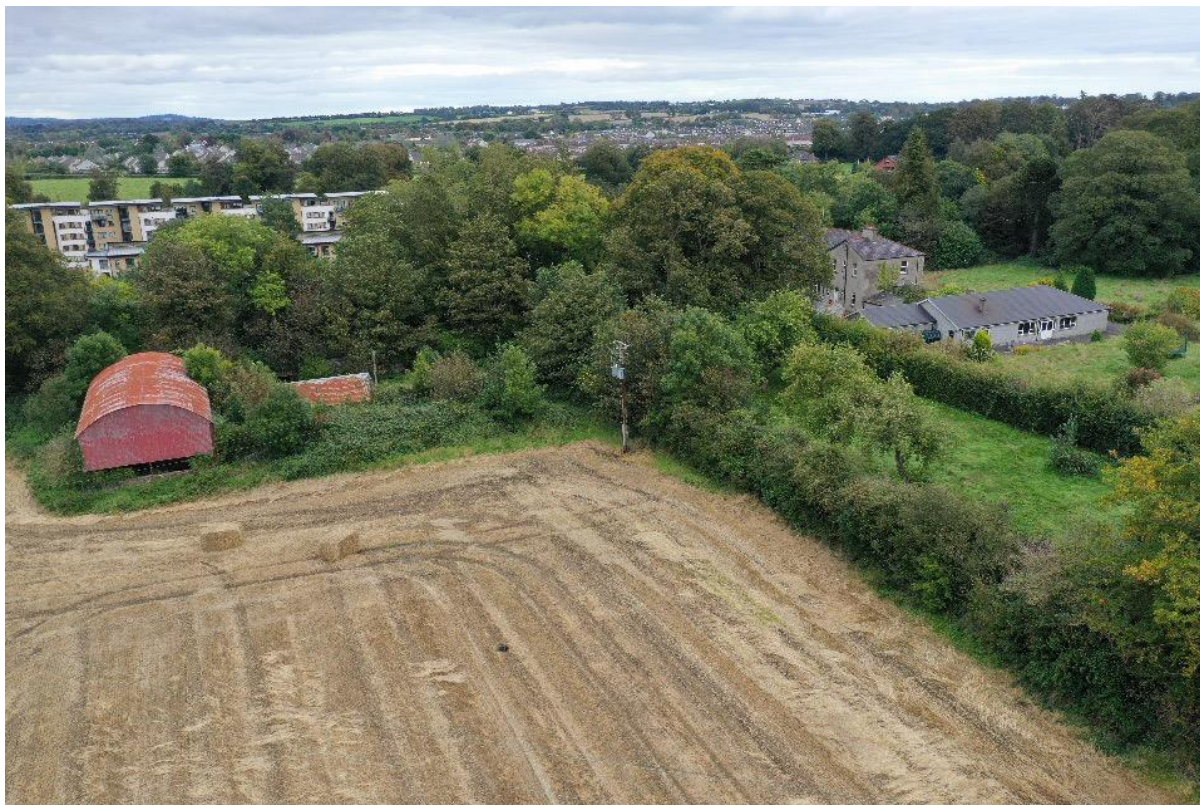
Plate 13.4.13: Aerial view of the former farmyard complex on the left of the photograph and Belmont House (partially screened by trees) on the right of the photograph. The single-storey farm building that was recorded by the NIAH is heavily overgrown
